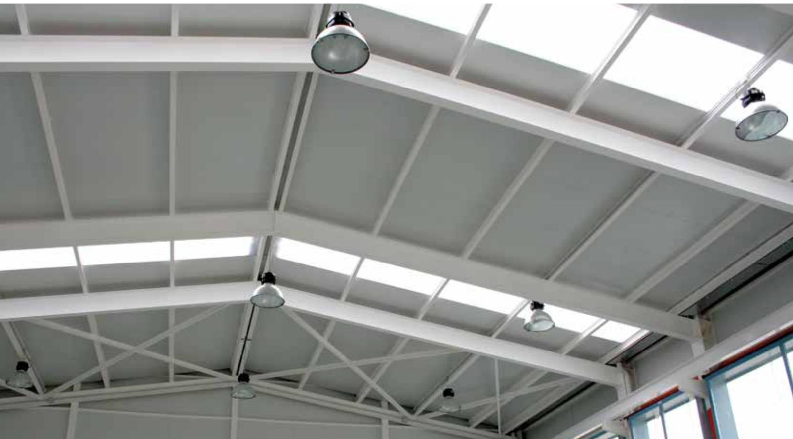
This is a perfectly waterproof solution, 100% effective, providing total watertightness. Its composition makes it a product that has high mechanical strength and durability. Danpalon polycarbonate provides good thermal insulation and requires no special maintenance.
